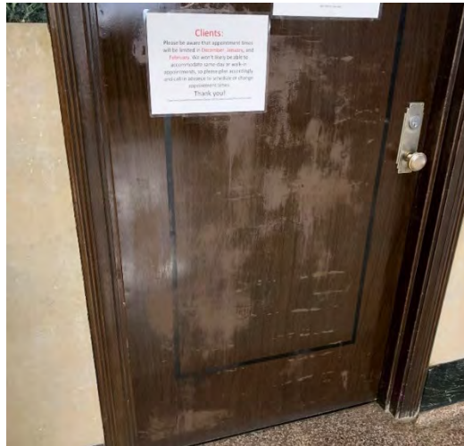
Figure 9: custom painted doors that will be repainted to match existing
