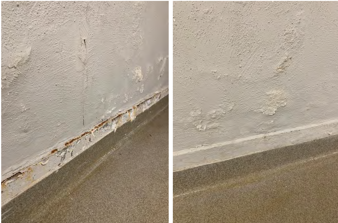
Figure 41-42: Water issues at the basement wall base: bubbling, cracking
