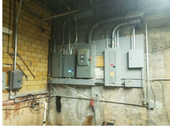
Figure 17 Main Electrical Gear
