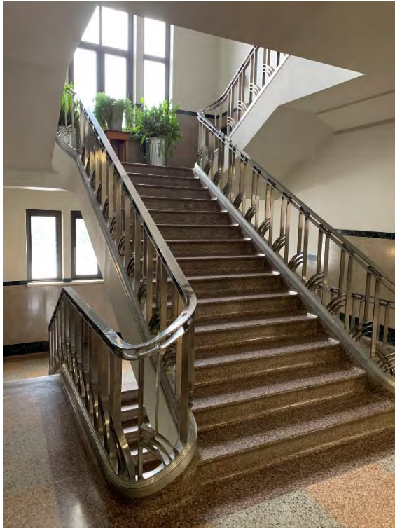
Figure 43: stairwell with original handrail
