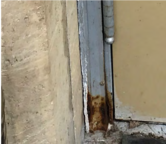
Figure 8: rusted door hinge at North door
