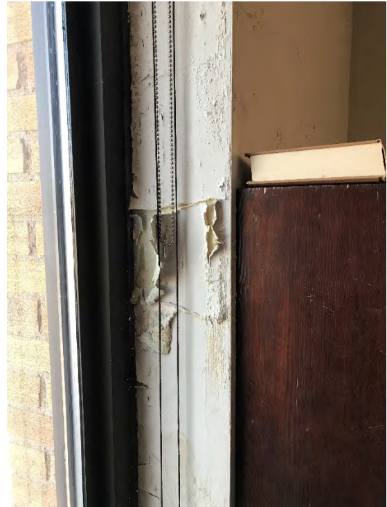
Figure 37: deteriorating finishes at the window in the evidence room, level 3
