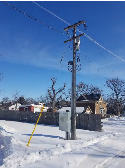
Figure 14 Existing Electrical Utility Transformer and C/T cabinet.
