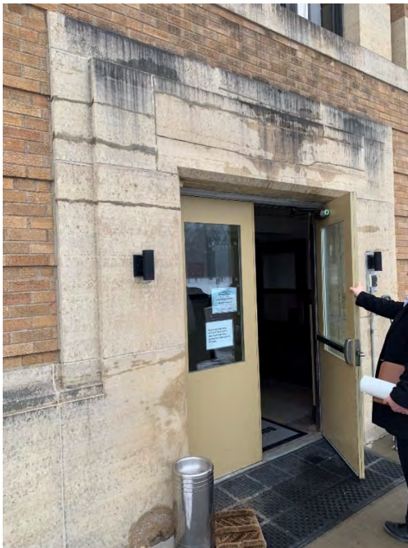
Figure 26: Water issues at stone lintel
