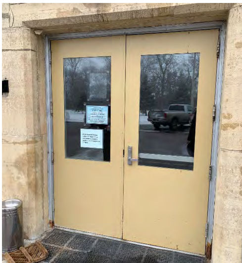
Figure 10: North set of exterior doors to be replaced
