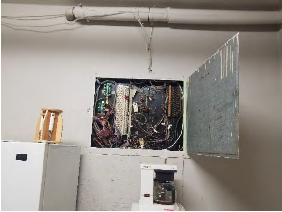
Figure 26 Old telephone wiring on basement floor
