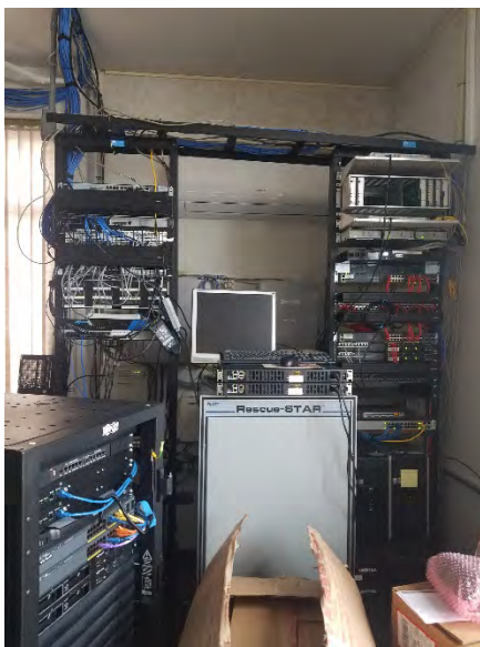
Figure 24 IT/Telecom racks, equipment
