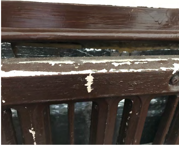
Figure 36: radiator paint chipping
