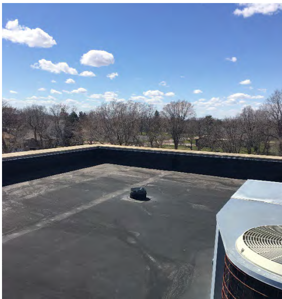
Figure 15: missing vent turbine
