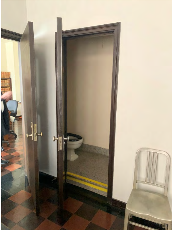
Figure 22: Step-up into 3 rd floor restroom
