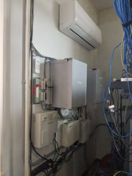
Figure 12 Indoor Wall Cooling Unit
