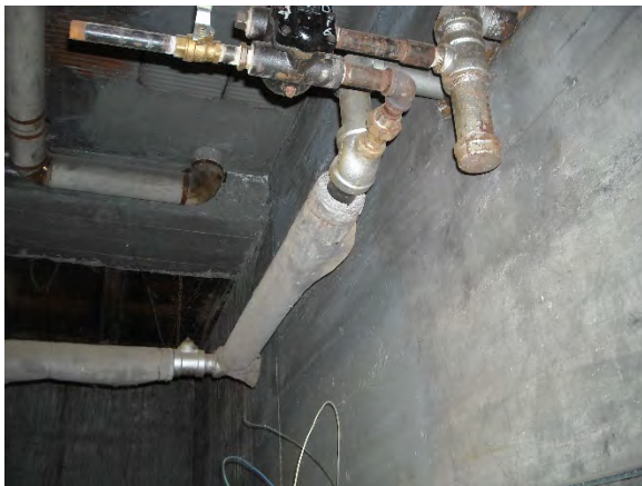
Figure 5 Steam Piping w/Asbestos Insulation
