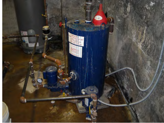
Figure 2 Condensate Return Unit
